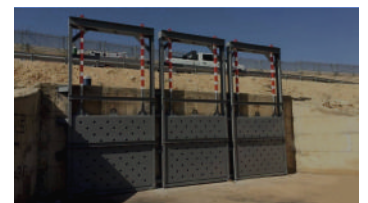
COUNTER INTRUSION GATE
