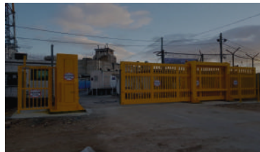
C400 SLIDING/CANTILEVER GATE RATING K4
