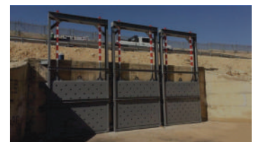
COUNTER INTRUSION GATE
