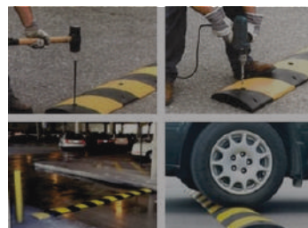
SPEED BUMPS AND PARKING RESTRICTORS
