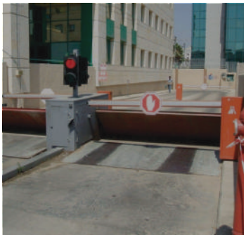
R500 SURFACE/SHALLOW FOUNDATION RATING K4
